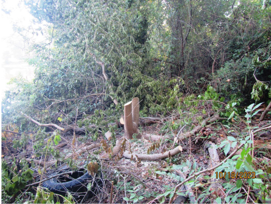
Photo 5. View of some partial clearing as seen by the remaining small tree trunks. Note some non-vegetative debris observed within the dense brush.
